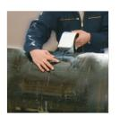
On smooth pipe surface which are in contact with the spacers (e.g. PE, PVC, steel/cast on PE-coated or stoneware) wrap a shear-secure-tape to guarantee an optimum security against slipping.
