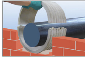
Connect half casings for fit until both halves rest on spacers
