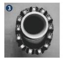
Slide belt assembly into annular space. For larger size belts, start inserting LINK-SEAL® modular seal assembly at the 6 o'clock position and work both sides up toward the 12 o'clock position in the annular space.
