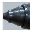
Pull sleeve tightly over the carrier pipe until the carrier pipe stands out clearly against the sleeve
