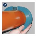
Please make sure that the cable or pipe is laying straight and centred in the wall opening. Put the two half shells of the PSI Sealing Plug around the cable or pipe and push the sealing in the opening. Attention: both half shells must be correctly positioned on each other. The plug must be pushed in until the flange touches the wall. Don't push any further!
