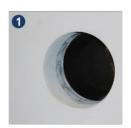
The wall opening (PVC sleeve, core drilled hole, steel sleeves....) must be cleaned inside. Please make sure that there is no dirt
